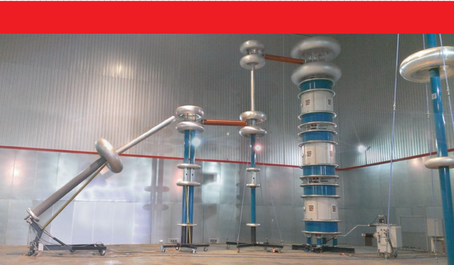
Fig. 2 Shielded room SSC 35x26x17 (incl. optional features) with integrated AC resonant test system WRM 5570/800 for type testing of high-voltage cables
